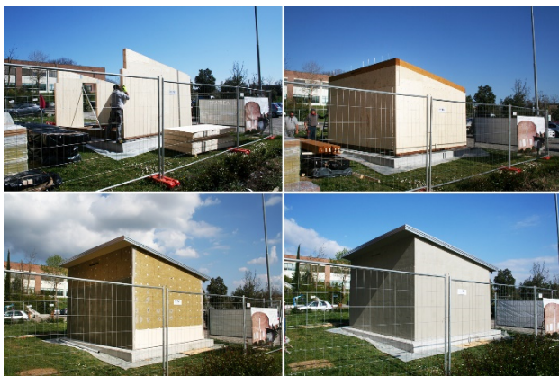
Figure 3. Different construction phases of the test room.
