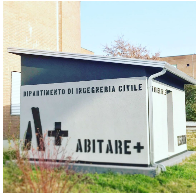
Figure 4. The completed test room.
