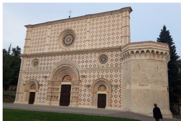
Figure 4. The Collemaggio Basilica in L'Aquila, that was restored after the 2009 earthquake
