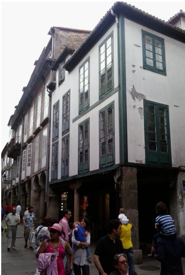
Figure 12. Houses with arcades in the Rúa Nova in Santiago de Compostela. An example of how the half timber typology evolved, conserving the arcade but increasing the façade openings and adding a floor. Source: A.F.P.
