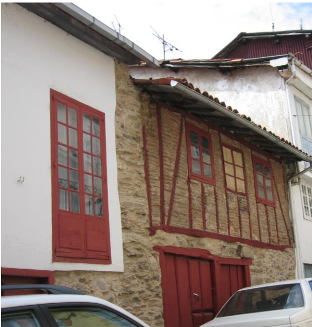
Figure 5. Houses of medieval origin with half-timbered walls with brick filling in Monforte de Lemos. The house on the left modified the facade openings at some later time. Source: A.F.P.
