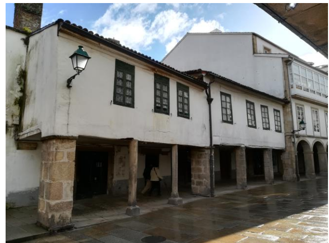
Figure 11. Houses with arcades in the Rúa Nova in Santiago de Compostela. One of the few preserved examples of housing typology with arcades and half-timbered structure with small holes. Source: A.F.P.
