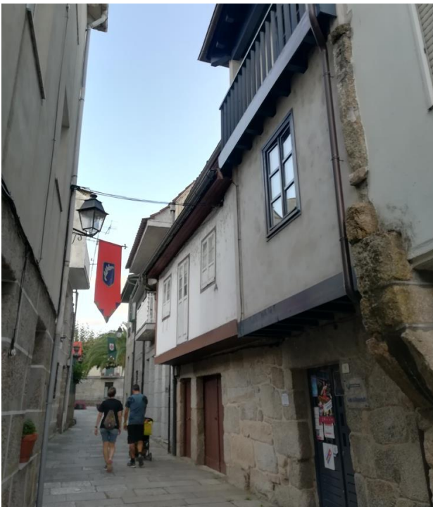
Figure 19. Cantilevered half-timbered houses in Ribadavia. Source: A.F.P.
