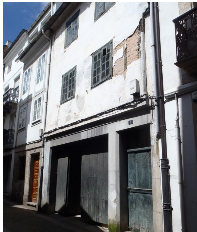
Figure 18. Half-timbered with brick house with a modified ground floor in Guevara street. Source: A.F.P.
