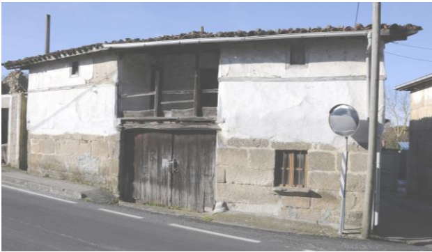
Figure 4. Rural house near the settlement of Maceda with half-timbered with earth floor. Source: A.F.P.
