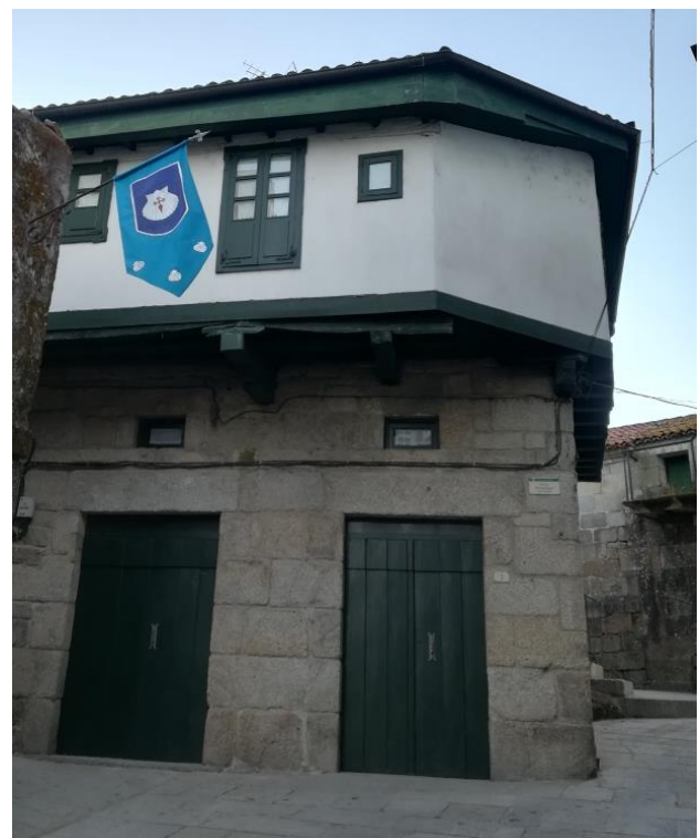
Figure 3. Medieval typology house in the city of Ribadavia, with a ground floor of stone and a half-timbered with earth first floor. Source: A.F.P.
