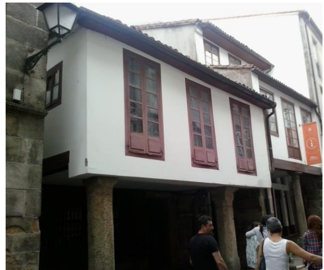
Figure 13. Housing with arcades in the Rúa Nova in Santiago de Compostela. Another example of how the timber frame typology evolved, conserving the arcade but increasing the façade openings. Source: A.F.P.
