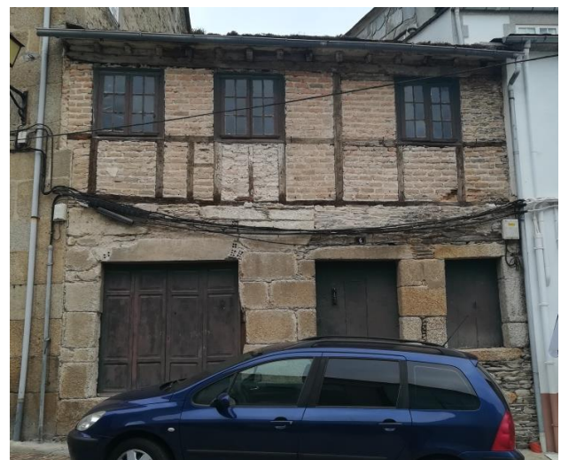
Figure 14. One of the examples of a medieval half-timbered house with brick filling and a stone ground floor that preserves the openings in the façade without modifying it. Source: A.F.P.
