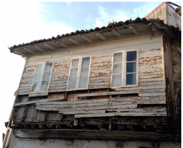
Figure 7. Half-timbered house with plank covering in Muros. Source: Muros City Council Rehabilitation Office
