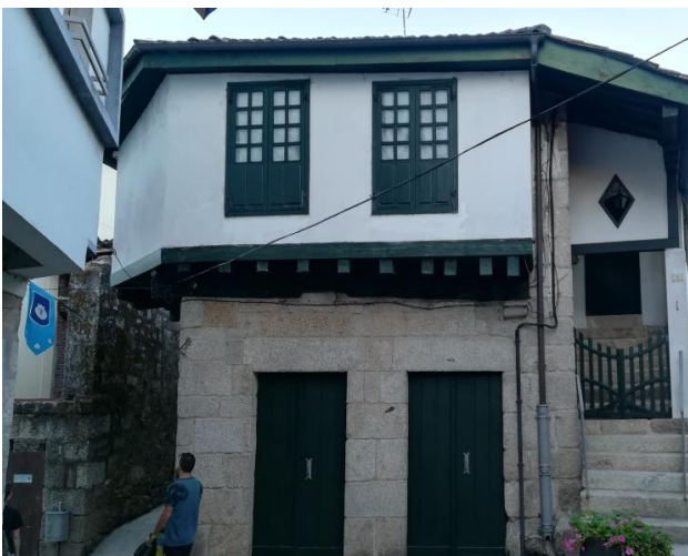
Figure 9. Half-timbered house filled with earth filling in the city of Ribadavia. Source: A.F.P.
