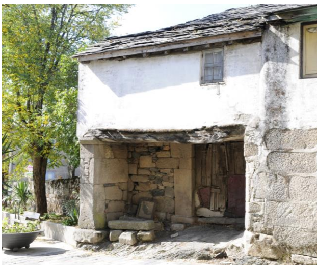
Figure 2. Medieval typology house with stone ground floor and half-timbered floor in A Gudiña settlement located on the Santiago route from the south. Source: A.F.P.
