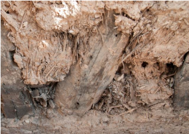
Figure 8. Detail of the half-timbered wall with earth in a house in Ourense. Source: A.F.P.
