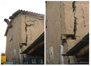
Figure 8. Crack in a furnace in Panguesillo, associated to poor links within its horizontal wooden reinforcement.
