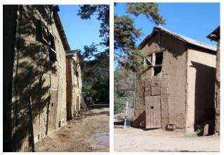
Figure 10. Severe deformation of a tabique wall associated with an inappropriate choice of wooden joints in pillars - Furnace in El Boldo.
