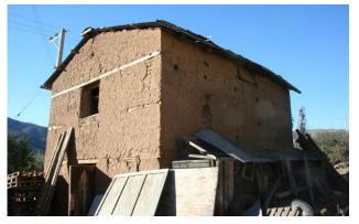
Figure 3. Adobe furnace in Chuchiñí, in which both continuous and corner horizontal wooden reinforcements can be identified.
