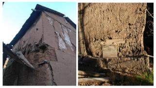
Figure 9a. Erosion in a. upper area of an adobe wall in Chalinga b. lower area of an adobe wall in Chuchiñi.
