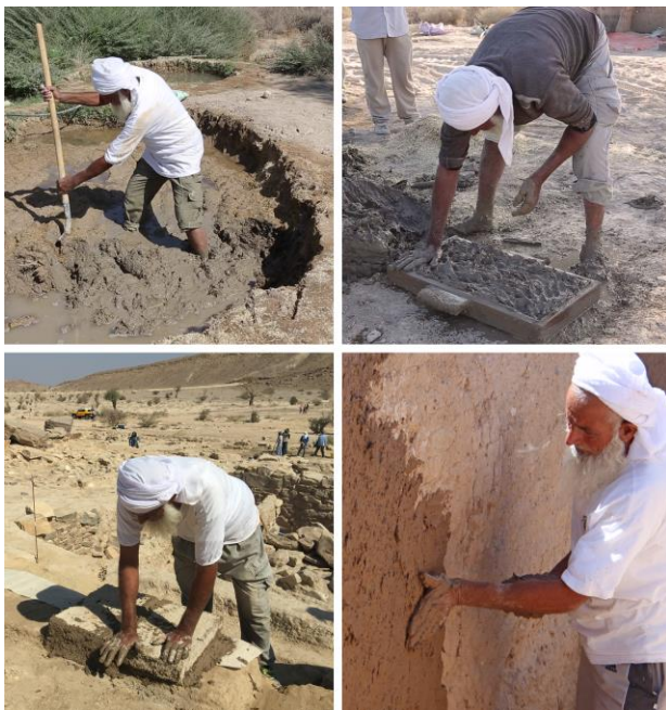
Figure 4. Mudbricks preparation, laying and wall plastering.
