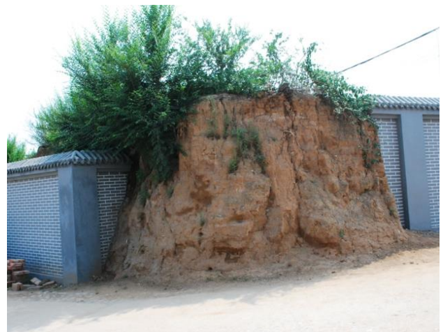
Figure 8. Present situation of human construction damage of the east town wall.
