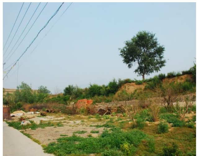
Figure 7. Present situation of plant diseases on the north town wall.
