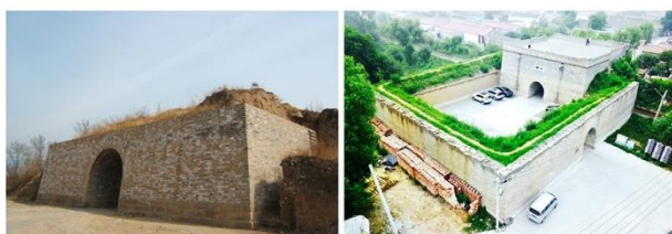
Figure 9. Comparison before and after the repair of the north town gate.
