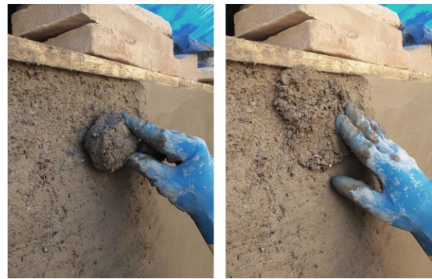
Figure 11. Surface reintegration with clay lumps, applied in the base and the final layer, by manual shaping and mashing.
