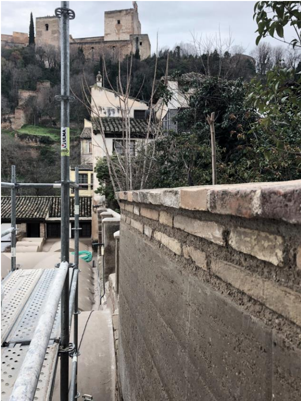
Figure 13. Courses and brick coping as upper auction of the rammed earth wall. At the bottom: the Alhambra of Granada.
