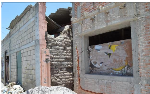
Figure 4. Adobe traditional dwelling with several modifications after the 2017 Puebla earthquake in Jojutla de Juárez, Morelos. Photo: Adrià Sánchez Calvillo (2018). © SPOT Image Copyright 2020.
