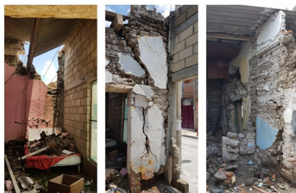
Figure 6. Damages in adobe buildings of Jojutla de Juárez. Photo: Adrià Sánchez Calvillo (2018). © SPOT Image Copyright 2020.
