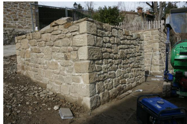
Figure 9. The new building under construction.
