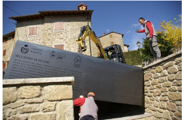
Figure 12. The monobloc of the COR-TEN ladder during the installation operations.
