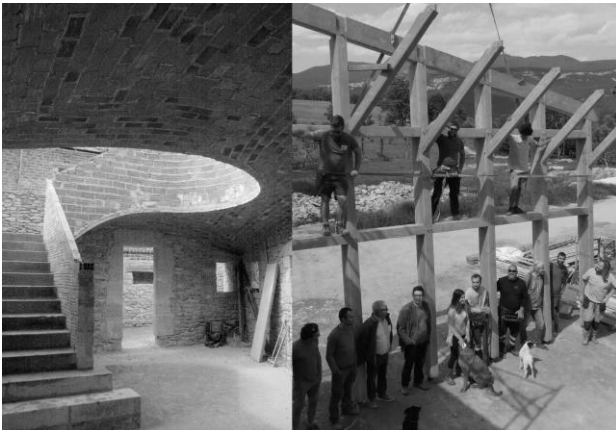
Figure 9. Catalan vaulting and massive wooden frame, two traditional techniques that allow the artisans to show their skills
