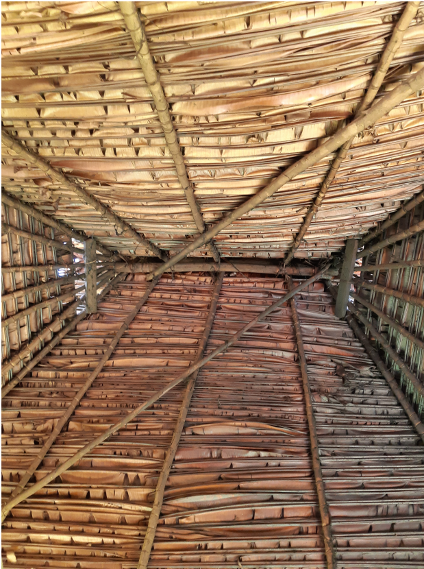
Figure 7. Bottom-up view of the inner roof made with Suita leafs. Santa María, Bonanza (Nathalia González).
