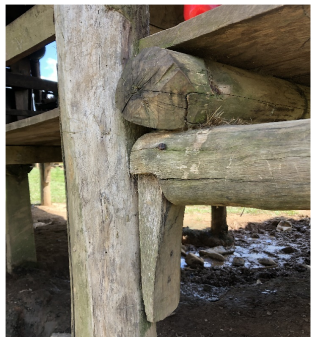
Figure 5. Detail of the structure of the main slab. Santa María, Bonanza (Nathalia González).
