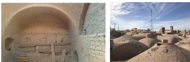
Figure 10. The material of adobe and straw-clay in these houses.
