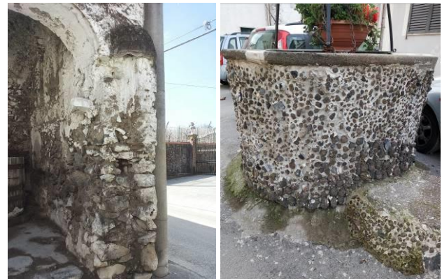
Figure 21. Lava masonry and water well (Boccia al Mauro, Terzigno).
