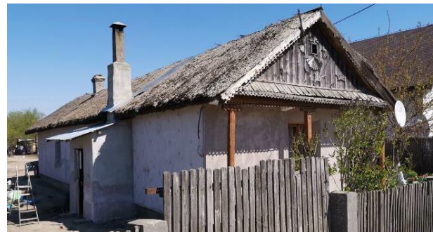
Figure 11. “Thermal rehabilitation” of an adobe house, in Sarichioi.
