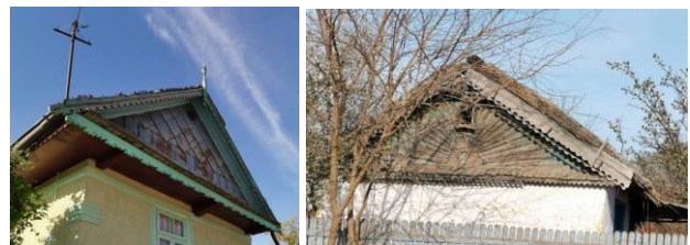
Figure 9. Gable decorated with metal shingles (left) or wood (right).
