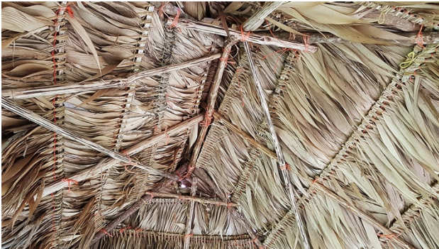
Figure 10. Oblique braces reinforcing the roof structure (Naso).
