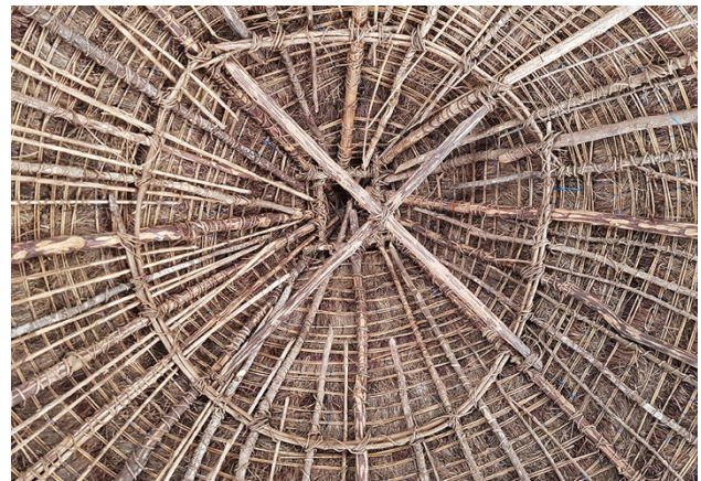
Figure 19. Roof structure of a Buglé building at El Peñón.
