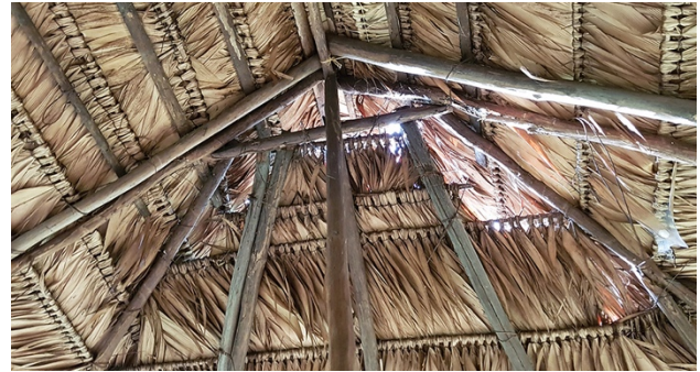
Figure 12. Free space at the upper end of the gable for ventilation, in a building in Guabo de Yorkin (Bribri area).
