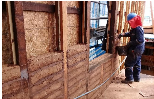
Figure 10. Installation of adobillo bricks.
