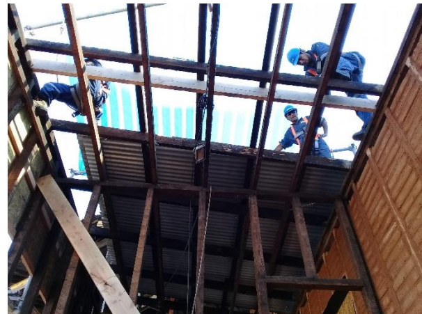
Figure 7. Structural consolidation of wooden beams.
