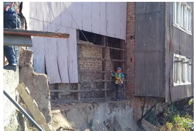
Figure 15. View of the wall discovered during restoration works.
