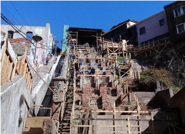
Figure 5. View of the railway at the Cordillera elevator.
