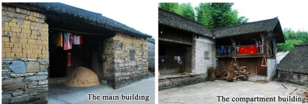
Figure 3. The main building and the compartment building.
