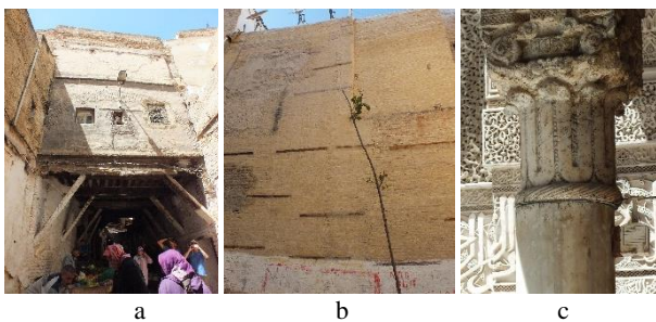
Figure 3. Some traditional anti-seismic techniques in Fes: a) covered passage with a discharging arc; b) wooden element in the masonry; c) “seismic isolator” in Attarine Medersa.
