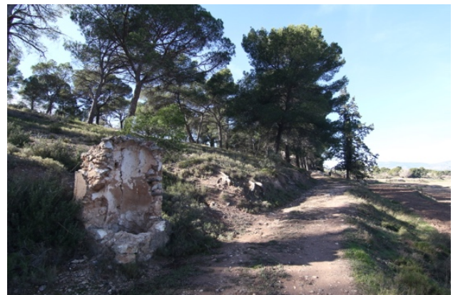
Figure 11. Cistern with a part of the top that protected the missing extraction system. The top, made of quarry stone with pargeting, was built with materials from the surrounding environment.
