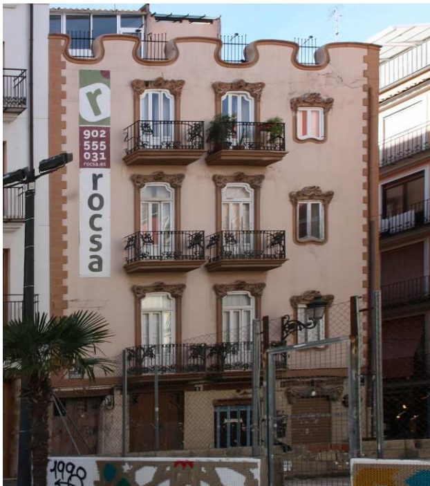
Figure 3. Facade. Casa Rotglà. Source: Own source.
