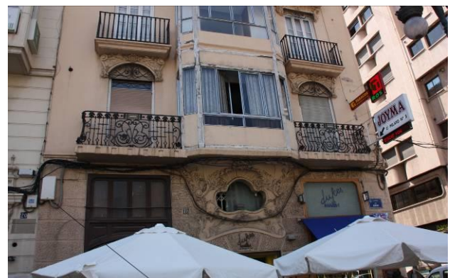
Figure 5. Facade. Casa Espert. Xativa Street. Source: Own photograph.
