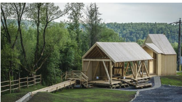
Figure 6. Sawmill, 2016. Zetea, Romania. Miklós Köllő, architect.
