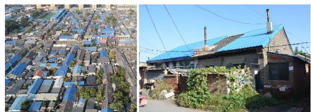
Figure 8. Traditional roofs covered by blue steel plates in the old town of Gaizhou. Source: Xing Zhenpeng and Li Bing, 2019.
