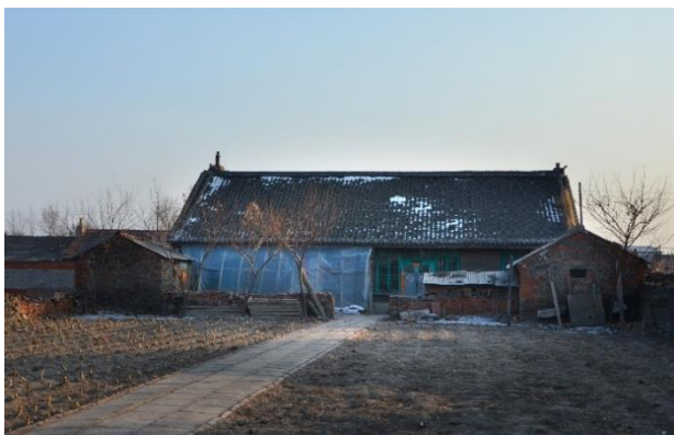
Figure 9. Walls covered with plastic film in the old town of Kaiyuan. Photo by Li Bing, 2017.
