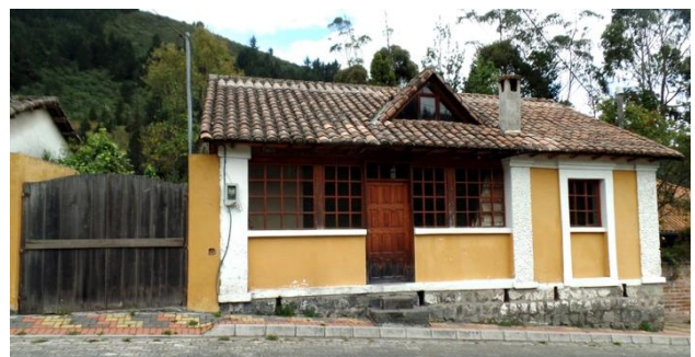
Figure 5. Continuous Opening type House, Nono, Ecuador, 2019.
