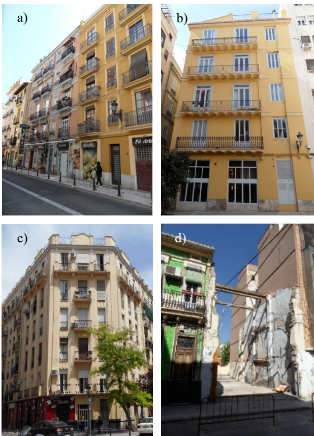
Figure 4. Aggregate building position; a) middle, b) corner, c) header, d) adjacent to a long-term empty plot (credit: the authors).
