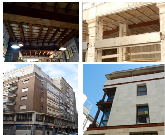
Figure 16. Example of structural typologies in Valencia: URM timber beams and joists; URM steel beams and joists, Reinforce concrete and Steel structures (credit: the authors).
