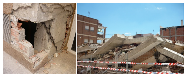
Figure 2. Buildings with short columns after Lorca 11th May 2011 earthquake (credit: the authors).
