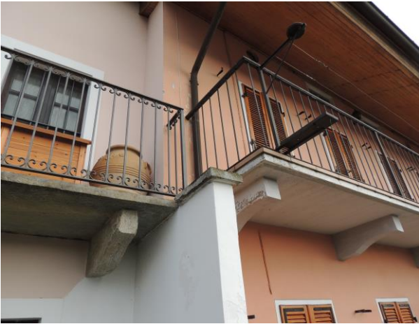
Figure 7. Building E - Balcony with reinforced concrete structure (credits Fabio Fratini).
