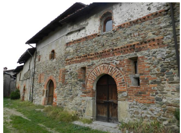
Figure 17. Building H - Preservation of the surface of the external wall and of the access portal (credits Silvia Rescic).
