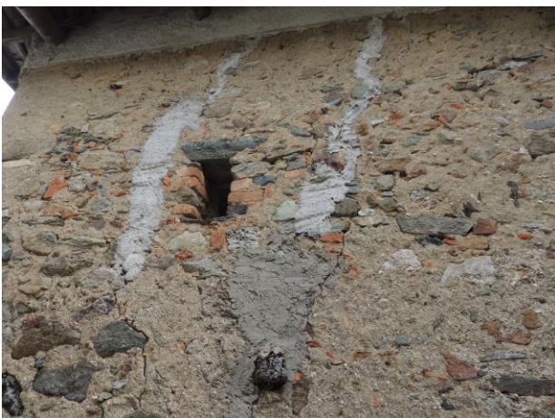
Figure 15. Building G - Filling of cracks with cement mortar (credits Fabio Fratini).
