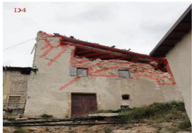
Figure 6. Structural Unite #165. Damage class D4 is assigned (EMS98).
