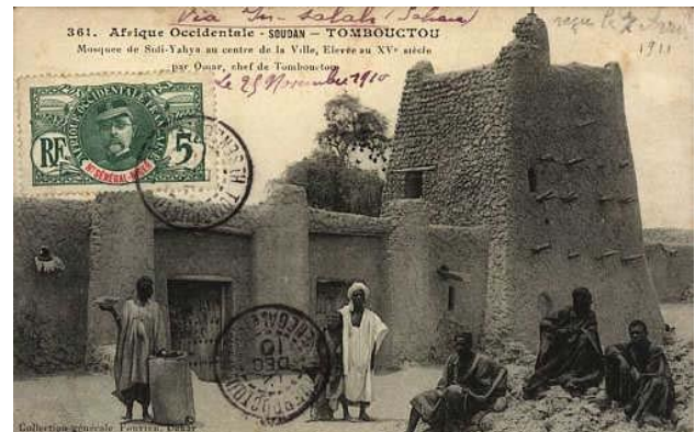
Figure 11. Postcard sent on 25 November 1910 showing Sidi Yahia Mosque with serious erosion of the eastern elevation of its minaret. (Collection Fortier – archives MCT).
