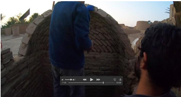
Figure 3. Excerpt of a video of a master builder in the process of constructing a barrel vault without centring, Esfahak, September 2019.
