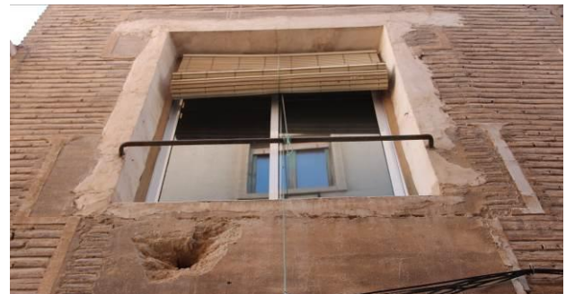
Figure 16. Mixed rammed earth wall on calle Caño no. 17 (Source: authors).
