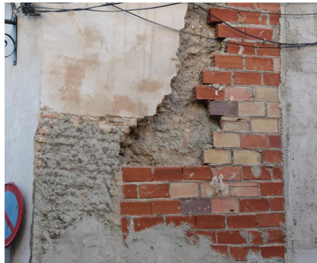
Figure 17. Hollow brick layer added to a rammed earth wall (Source: authors).
