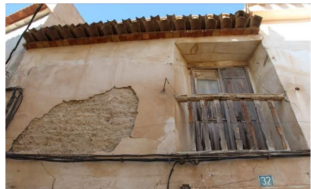
Figure 7. Simple rammed earth wall rendered with gypsum (Source: authors).
