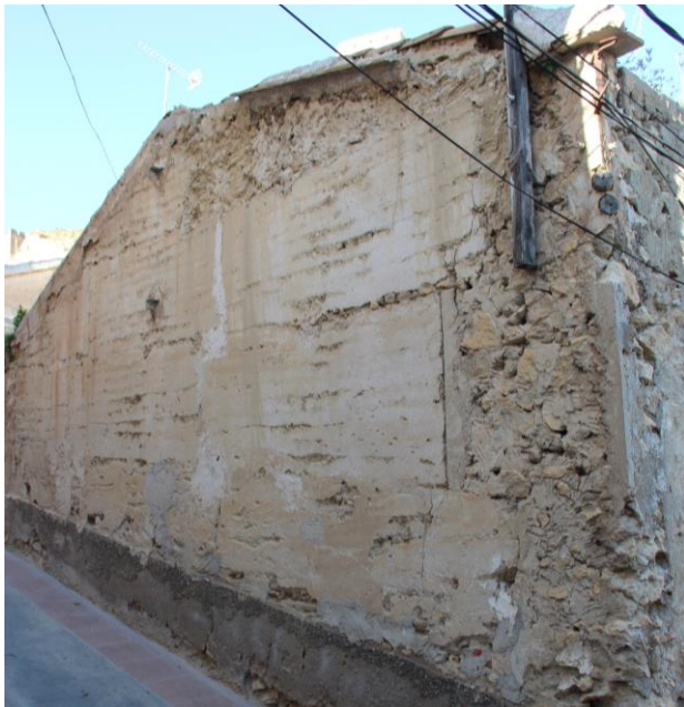
Figure 9. Gypsum-crusted rammed earth wall and gypsum guided masonry pillars (Source: authors).
