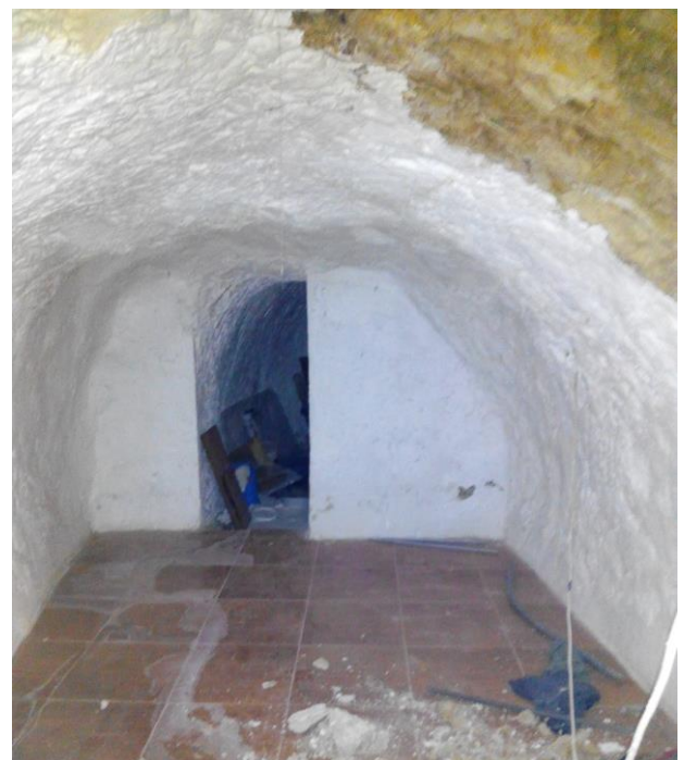
Figures 12. Detail of the interior of the casón on calle Mizas no. 41 (Source: Mula Town Council).
