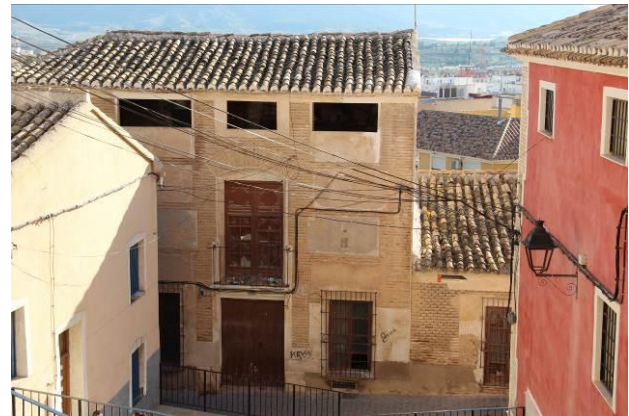
Figure 10. Mixed rammed earth wall in the dwelling on calle Sastres no.7 (Source: authors).
