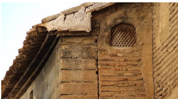
Figure 14. Rammed earth corner supplemented with bricks (Source: authors).
