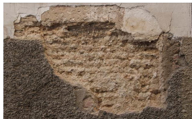
Figure 8. Detail of the lime layers of a lime-crustrated rammed earth wall (Source: authors).
