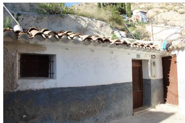
Figure 11. Exterior of the casón on calle Mizas no. 41, exterior and detail of the interior (Source: authors).
