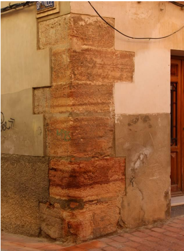
Figure 13. Detail of an Almagra stone corner plinth in Mula (Source: authors).
