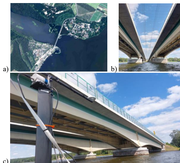
Figure 1. Bridge over Lake Zegrze a) orthophoto (GSD = 5 cm), www.geoportal.gov.pl ; b) bottom view; c) side view
