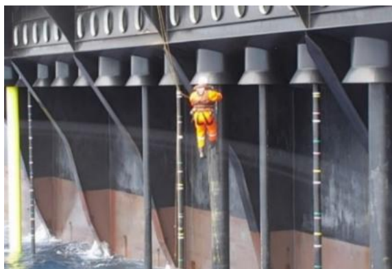
Figure 1- Rope-access riser inspection (Buschinelli et al., 2020).
