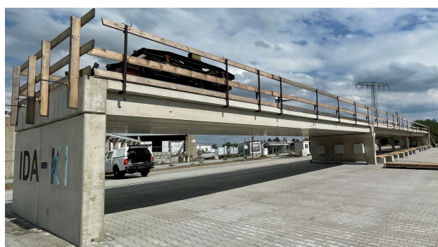
Figure 1. IDA-KI openLAB research bridge with load vehicle.
