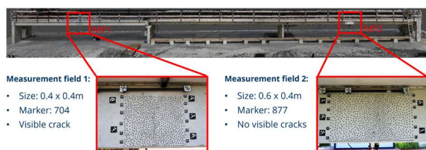
Figure 3. Installed photogrammetric measurement fields and their locations on the openLAB bridge.
