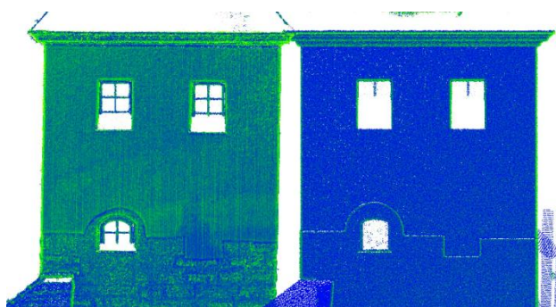
Figure 12. Close-up roughness comparison of the tower façade.
