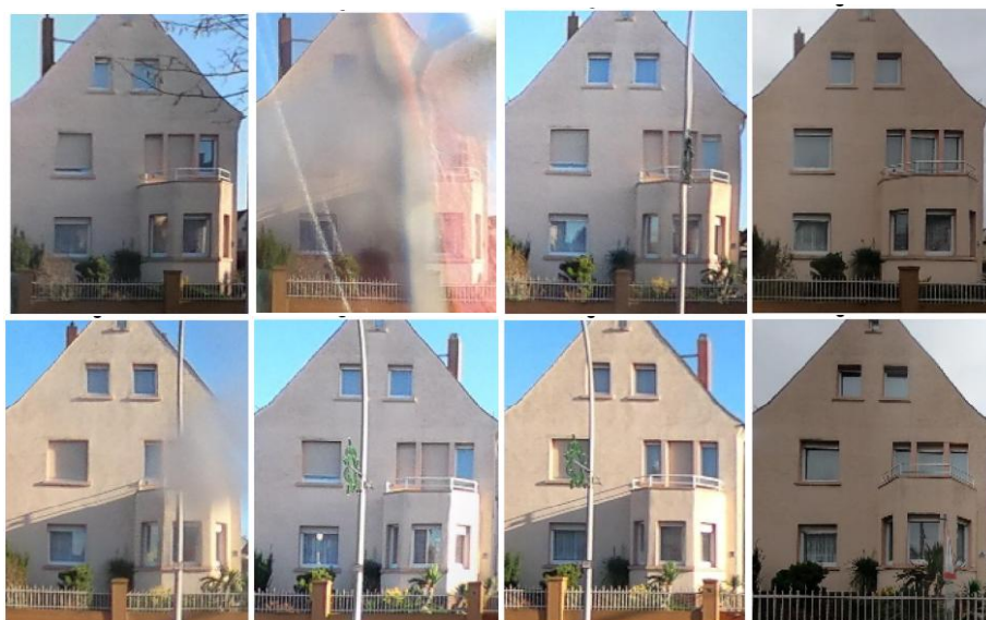
Figure 3. Rectified (normalized) façade images for all selected camera stations shown in Figure 2c. Perspective distortions are removed through façade-based rectification, resulting in fronto-parallel views. Some images exhibit occlusions (e.g., trees or street objects) and motion blur, reflecting the challenges of unstructured image acquisition.
