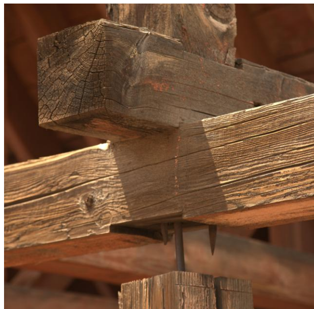
Figure 12. Withdrawn joint from Pioche Mine
