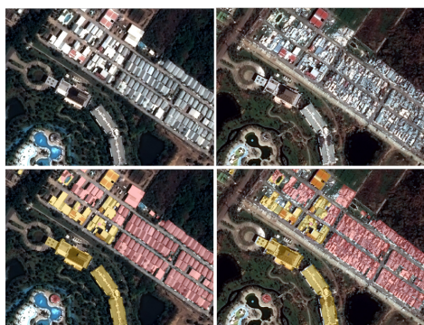
Figure 9. Building damage assessment on Acapulco. Top: Pre-event and post-event images; Bottom: Predictions (red destroyed, orange damaged). Pléiades ©CNES 2023, Distribution CNES PWH.
