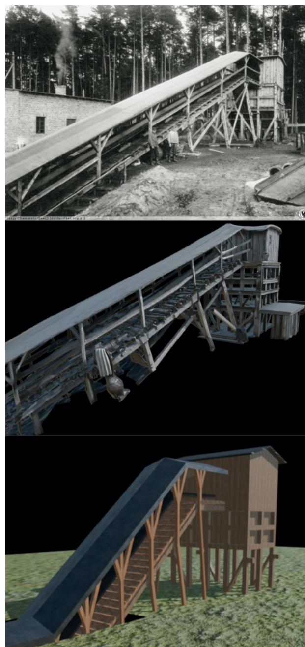
Figure 11. Archive photo of the above-ground structure of the inclined conveyor system (top), AI-reconstructed 3D model (middle), and manually reconstructed model (bottom).
