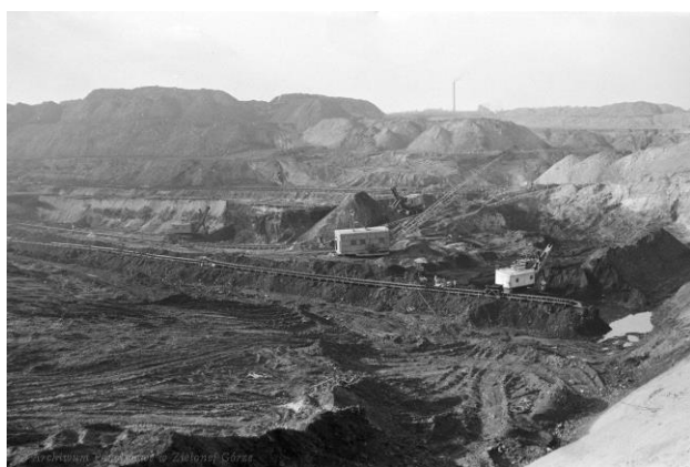
Figure 1. Part of the open-pit in the "Przyjaźń Narodów - Szyb Babina" mine ca. 1964-1967 (photo by Cz. Luniewicz, source: National Archive in Zielona Gora, Poland)
