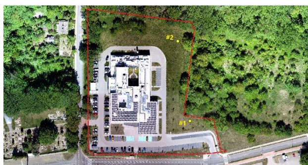
Figure 1. The analysed cadastral parcel (outlined with a red dashed line) with the two considered antenna locations (indicated #1 and #2).
