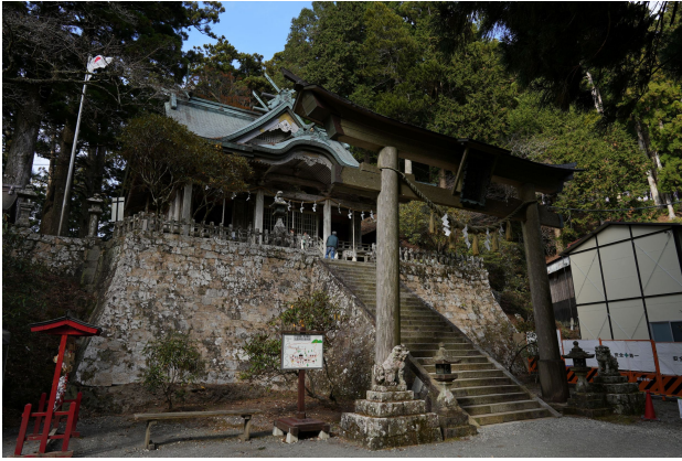
Figure 1. Main hall of Tamaki Shrine
