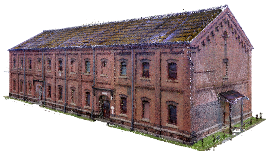
Figure 7. External view of the Red Brick Storehouse visualized by SPBR.
