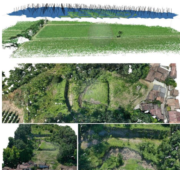
Figure 1. Images of the two case studies analysed in this phase of the ongoing research: above, plain of Pavia in Po valley; below, Oltrepo' Pavese landslide.
