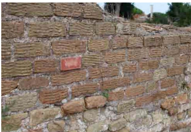
Figure 2. Restoration in Guild Temple with a small plaque with restoration year and scratched bricks [Rinaldi, 2012]
