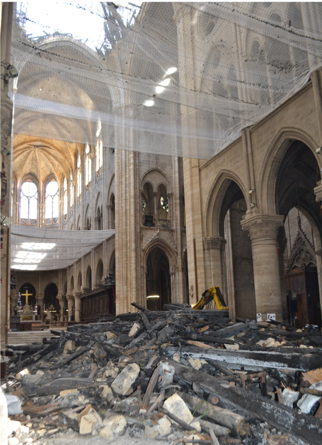
Figure 1: Examples of pictures taken in the context of a restoration site. Top: A pallet of debris (Claudine Loisel / LRMH) Bottom: The debris in the nave of the Notre-Dame cathedral (Aurélia Azéma / LRMH)
