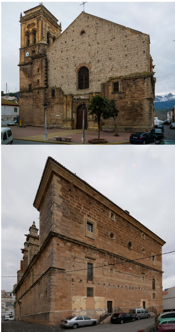
Figure 1. Main and back façade of the church of Nuestra Señora de los Remedios, Iznalloz.
