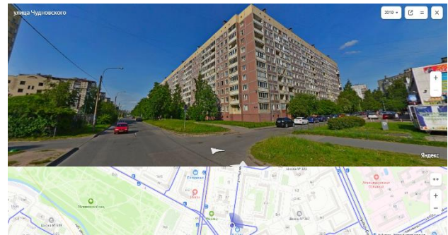
Figure 2. Overview image of buildings No. 8/1 and 8/2 on Chudnovsky Street.
