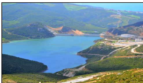
Figure 1. Tanger-Med dam in the north of Morocco.
