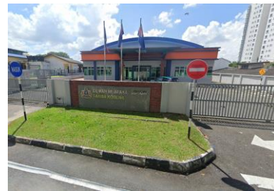
Figure 2. Front view of Dewan Taman Kobena, Johor.
