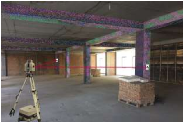
Figure 3. Spectral deformation zones of columns and floor beams
