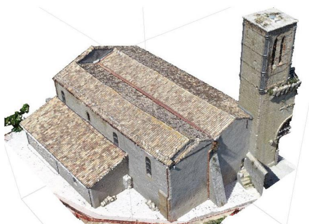
Figure 3. UAV digital survey and SfM point cloud.
