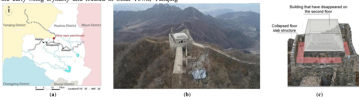
Figure 1. (a) Location of the Nine-eyes watchtower; (b) The status of the Nine-eyes watchtower; (c) The collapsed parts of the Nine-eyes watchtower.
