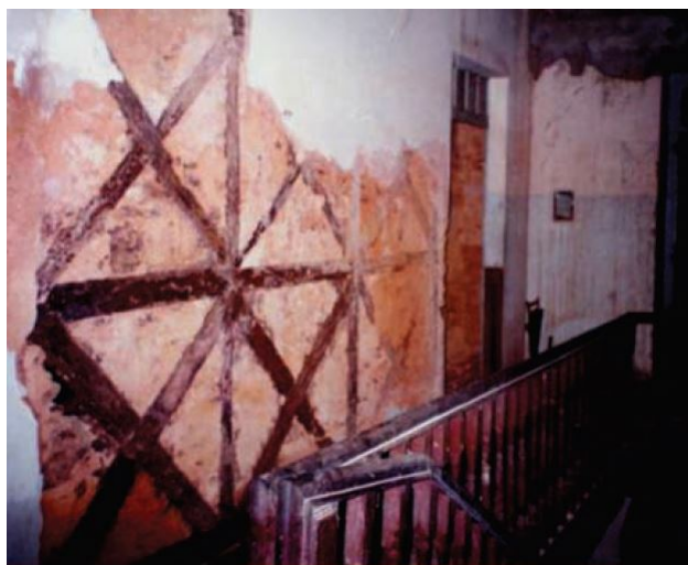
Figure 5. Wall evidencing the Santo André cross structure. (Figueiredo et al., 2011)
